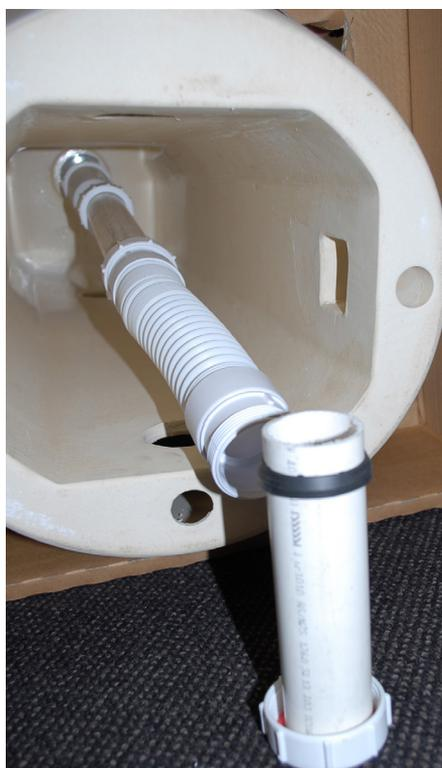
Fig. 3: Access under basin showing connection of flexible waste hose (provided) to 40mm PVC DWV in floor
