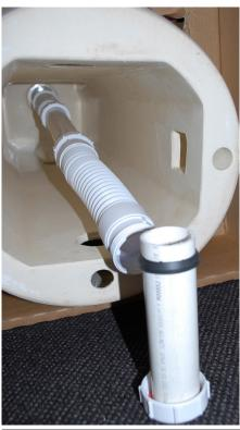
Fig. 3: Access under basin showing connection of flexible waste hose (provided) to 40mm PVC DWV in floor
