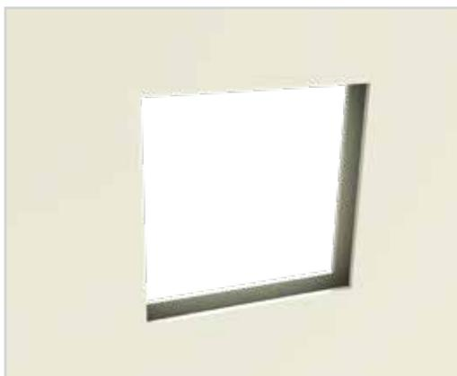
Mark and cut out hole the same size as the access panel. You can use the panel as the template. For a 600 x 600mm nominal APM, the ideal cutout size is 600 x 600mm.
