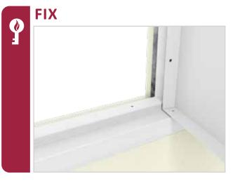
Fixings must be appropriate for the barrier- Min. 7g screws for framed wall.
