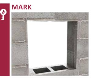
Mark and cut out hole the same size as the access panel. You can use the panel as the template.For a 600 x 600mm nominal APM, the ideal cutout size is 600 x 600mm.
