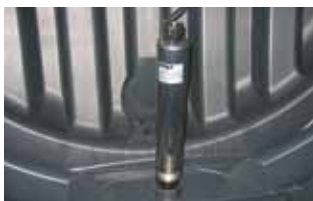
7. Insert pump into base of tank before connecting tank top
