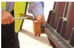
8. Hammer in quick connectors
