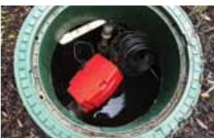
14. Install Graf filter and electrical connections
