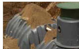
12. Backfill hole in 300mm layers, see page 1.
