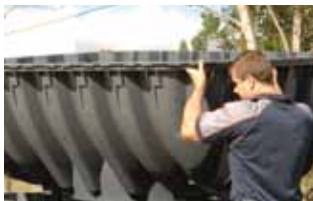
4. Lift tank in halves
