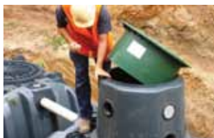
11. Push dome into position and lube seal with liquid soap provided. Then insert shaft.
