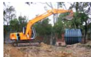
9. Lift tank into hole and recheck level
