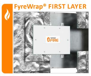
Install FyreWrap® Elite 1.5 according to FyreWrap® installation instructions, ensuring that the material fits snugly into the provided recess in the FWAP frame on all sides. See the FyreWRAP® Ductwork Technical Manual for more details.
