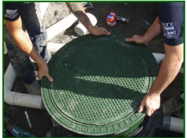
10. Install Graf Telescopic Shaft & Lid (man hole) to tank and complete landscaping
