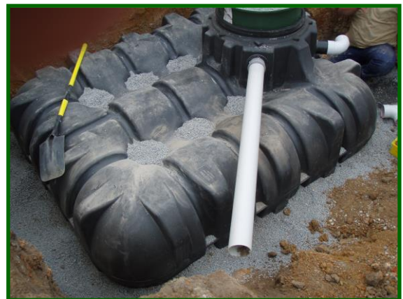
6. Connect plumbing, 1/3 fill tank with water and then back fill
