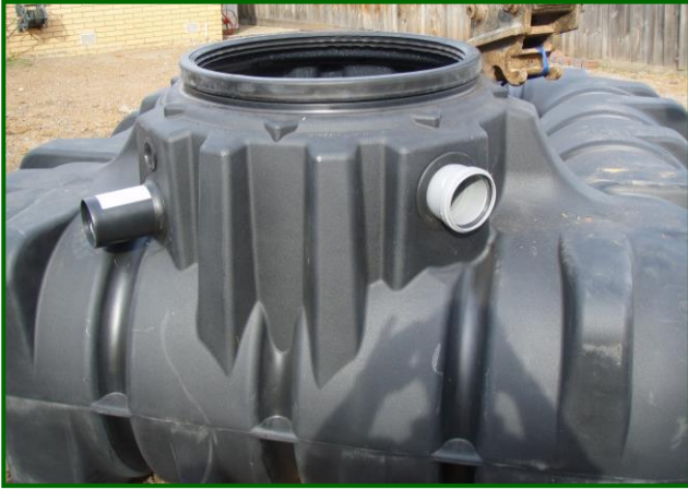
7. Insert tank seal and plumbing connection fittings
