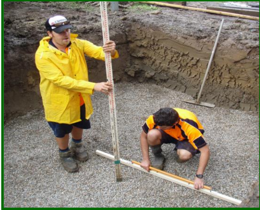
1. Dig excavation and provide 100-150mm well compacted level base
