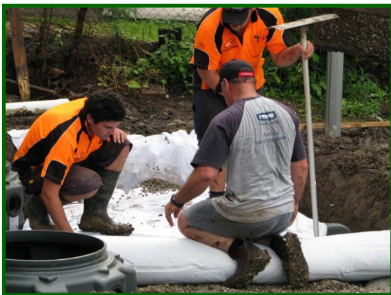
5. Install geotextile cloth over tank and ditch and up to ground level if ground water could be above the shoulder of the tank.
