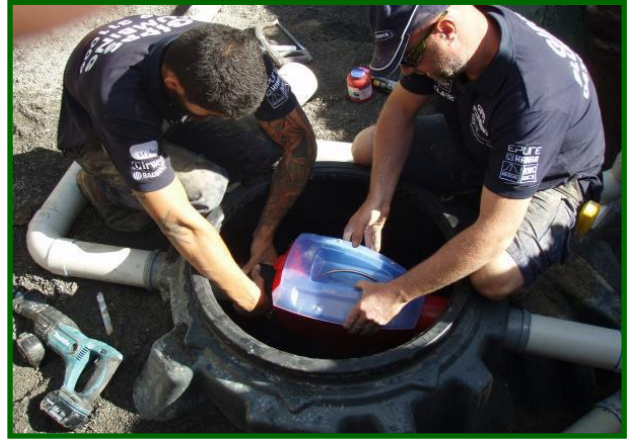
8. Connect Minimax Filter Package (see instructions pages 12-13)
