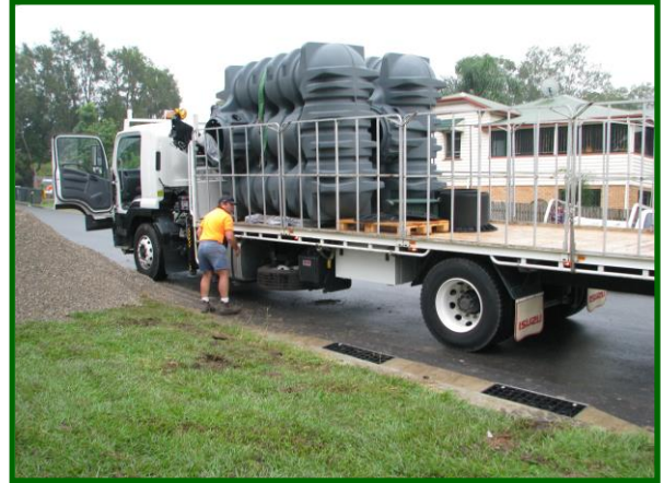
2. Lift tank/s off truck using suitable lifting equipment
