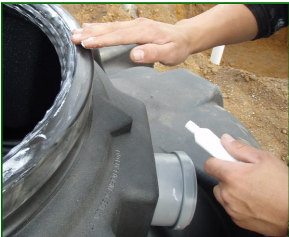
9. Lube up rubber seal with liquid soap provided before inserting Shaft & Lid
