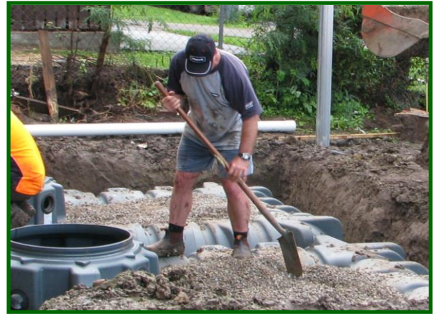
4. Back fill must be compactable porous with a maximum size of 7mm
