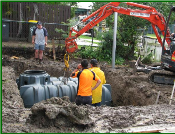
3. Use digger to lift tank/s into the hole
