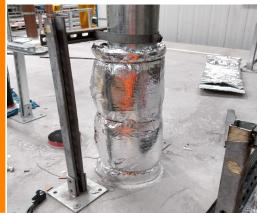
Floor penetrations require TWRAP<sup>M</sup> to be applied to the top side only, whereas wall penetrations require fire rating from both directions, so TWRAP<sup>M</sup> is required to both sides of the wall.
