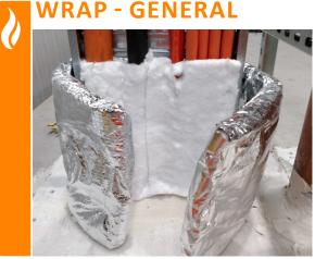
Wrap the TWRAP<sup>™</sup> around the service, ensuring there is a minimum 50mm overlap between any overlapping sections of wrap.
