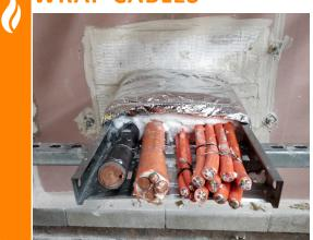
For cable tray penetrations, voids in the cable tray must be filled with loose TWRAP<sup>™</sup> infill material as shown in photo above (This is not required for bundles of cables not installed on cable trays).
