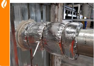
Strap in place with minimum 4.6mm wide steel cable ties, every 150mm and at every overlap where you are using more than one width of TWRAP<sup>™</sup>. Cable ties may be joined to create longer ties.
