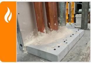
Apply FyreFLEX® Sealant to the full depth of the FyreBOARD Maxilite®, then finish with a 50x50mm fillet.
