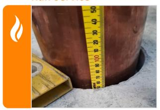
Form the correct sized hole per the approval's tables above, then the service can be run through the concrete slab.
