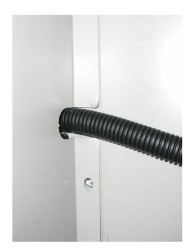
Step 16 remove the tab on the side of the electrical entry to the heat pump module
