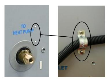
Step 4 connect wiring and secure conduit with saddle clamp
