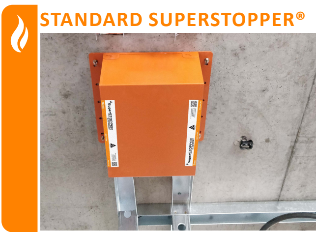
SuperSTOPPER® top plate, body and approved services all installed as standard to the soffit, with foam end plugs installed around the services.
