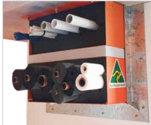
Where a large run of services needs firestopping in a small width of wall
