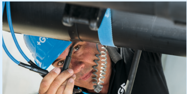
Connect the welding cables to the welding contacts of the fitting and weld according to the instruction manual.
