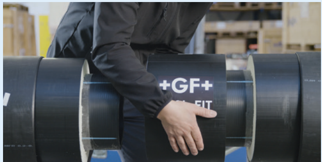
Slide-on the shrink sleeves and push the pipe ends up to the stop into the electrofusion coupler.
