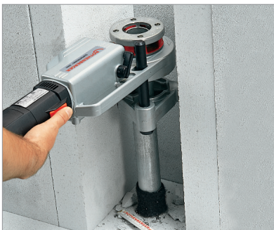
Work in confined spaces
