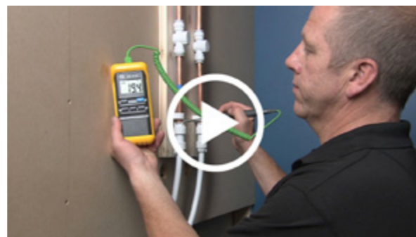
Perform cold water isolation test
