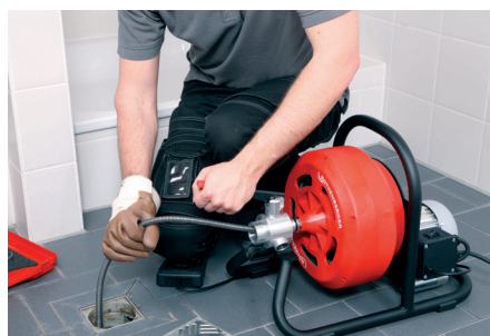
Cleaning of floor drain with 13 mm spiral
