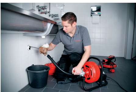
Cleaning of connection pipe with 10 mm spiral
