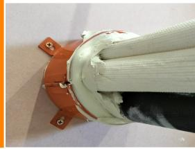
Use appropriate fixings as per page 8 to secure the collar to the wall/floor using all of the available the fixing tabs.
