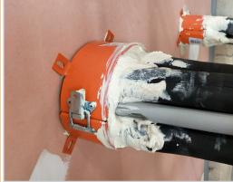
Fit the FyreCHOKE Premium Hinged Retrofit Collar, undo the latch to open the collar, secure it around the service/s, and re-secure the latch.
