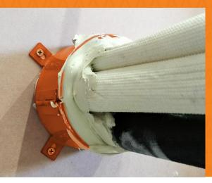
Trafalgar Fire is proud to present our newly developed Mixed Service Collar approvals for HVAC&R penetrations with our FyreCHOKE mixed service collar. Treat multiple sets of pair coil plus their cables, insulated pipes and drain lines all through one penetration, making HVAC&R penetrations fast, clean and easy.
