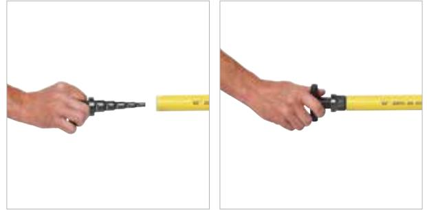
7. Insert the approved calibrating/deburring tool into the pipe, and then alternately turn in a clockwise and in a counter-clockwise direction. Ensure that a consistent, smooth chamfer is formed on the end of the pipe.
