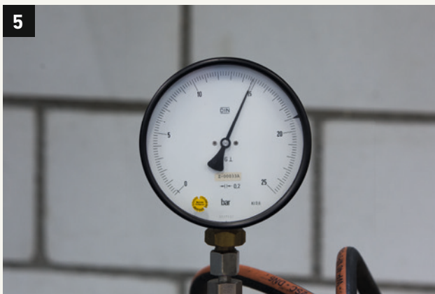
5 Check the system with a pressure test.
