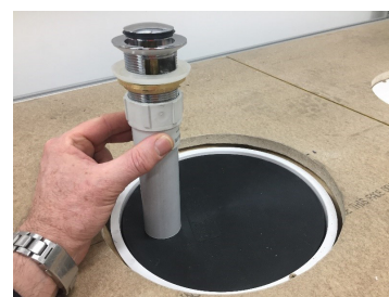
Waste pipe into smart seal
