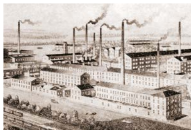
FIRST MECHANICAL FACTORY FOR SANITARY WARE ON THE EUROPEAN CONTINENT, ZNOJMO
