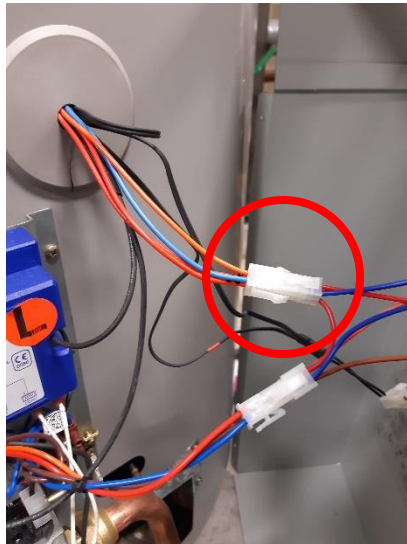
Unplug Molex plug that is run from water heater jacket
