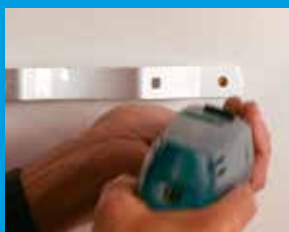
Step 2 – Position bracket and fasten to wall.
