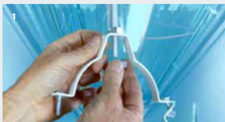
Step 1 – Trim All Thread to required length. Measure and mark off fall line and screw the first locating nut above this position.
