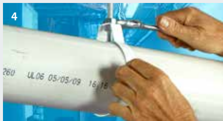
Step 4 – Fit remaining pipe and make any minor pipe fall adjustments prior to tightening off.
