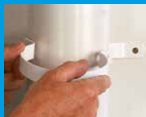
Step 3 – Place pipe into bracket base.
