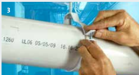
Step 3 – Secure the lower section with the hi-tensile, zinc plated bolts and nuts (supplied).
