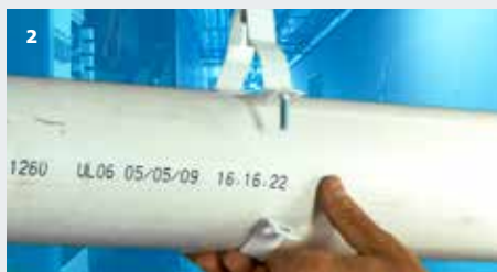
Step 2 – Position bracket and swing lower section out of the way and fit pipe.
