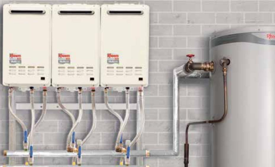
Manifolded banks of Continuous Flow Water Heaters (CFWH) meet the peak demand period requirements whilst the storage tank provides buffer for peak simultaneous demands.
