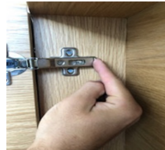
2. Push down clip and remove door
