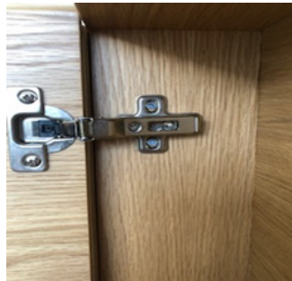
1. Loosen the 2 screws on each side and lift door up and down, re-tighten screws.
