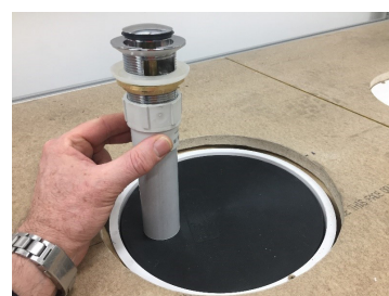
Waste pipe into smart seal
