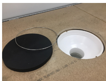
Below floor smart pan
