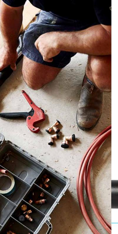
The Auspex Crimp System, made for both cold and hot water applications, has revolutionised pipe fitting with its 'cut, fit, crimp, done' process.
