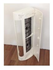
Remove the front facia from the wall mounted split system and clean.
