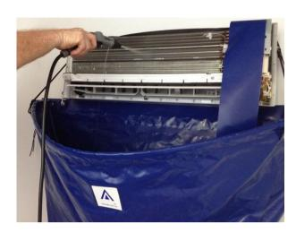
Cover the electrics with a plastic cover for protection. You can now pressure clean both the coil and drum fan.
