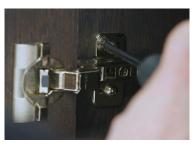
Turn screw found on the hinge mount. This can be turned left or right.
