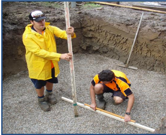
1. Dig excavation and provide 100-150mm of well compacted level base
