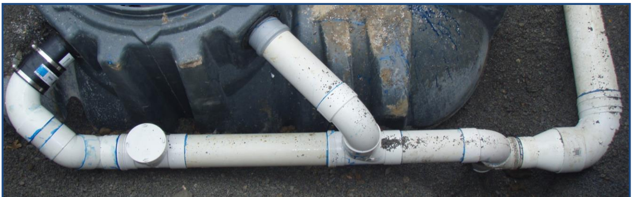
5. Connect plumbing, 1/3 fill tank with water and then back fill. Refer 5.3
