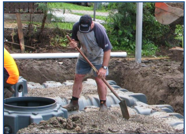
4. Back fill must be compactable porous with a maximum size of 7mm. Refer 5.3
