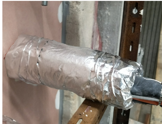
TWRAP secured on each side of penetration using three strips of reinforced aluminium tape applied around the wrap's circumference. TWRAP applied on both sides of the wall. Alternatively, apply steel ties 50mm from each end and at 150mm centres in between.
