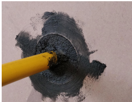
FyrePEX TM HP Sealant applied to full depth of plasterboard.
