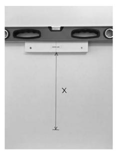
3. Locate the wall bracket using the dimension table below. Dimension X is the distance from the base mark A to the underside of the bracket. Suitable screws and wall fixings should be used to FIRMLY SECURE the bracket to the wall. <a href="IMPORTANT:">IMPORTANT:</a> the wall fixings chosen must accommodate the weight of the mirror.
