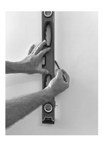
**2.** Using a level, plumb the centre line up the wall
