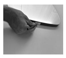
**1.** Place mirror in the desired position and mark the wall at position **A** shown on the base of the mirror.
