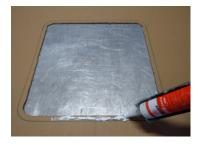
Place the sink into the benchtop, wipe away excess silicone, and leave to cure for 24 hours before use
