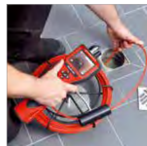
Inspection of floor drains
